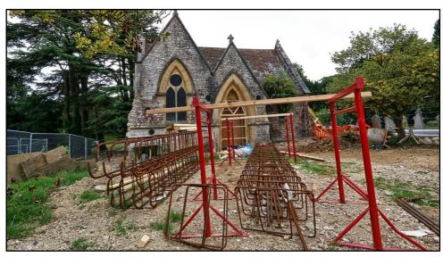
Work-in-Progress; it looks like a building site - and it is! The Contractors have been proceeding very well indeed preparing for the underpinning. 70 piles (35 pairs) are now inserted inside and outside the chapels; some of these are 15 metres long (ie: deep!). These will support beams on which the chapel structures will sit – planned by year-end.
